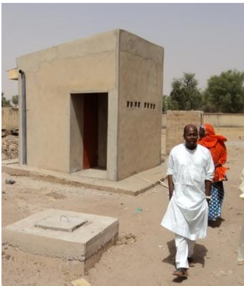
New VIP latrine under construction
