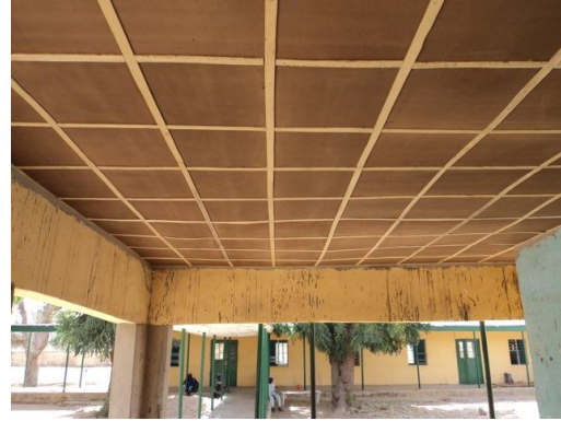
Ceiling reconstructed awaiting
