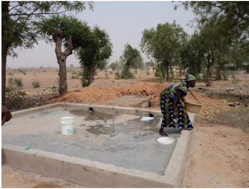
Laundry location with standpipe and good drainage (under construction)
